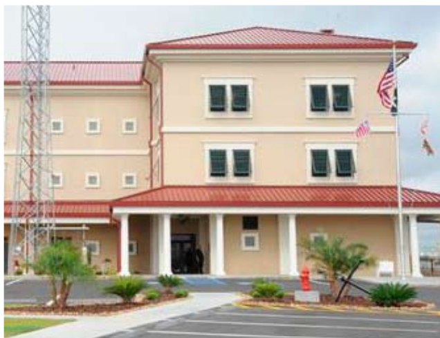
The old building destroyed by Hurricane Katrina, the new one is designed to withstand a Category 4 hurricane. U.S. Coast Guard photo
